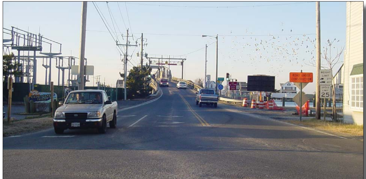
Old Bridge Area While Still in Service
