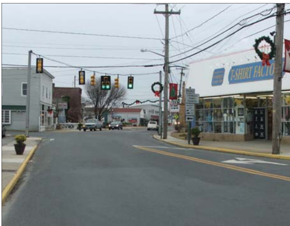
Existing Power Poles Along Main Street at Old Bridge
