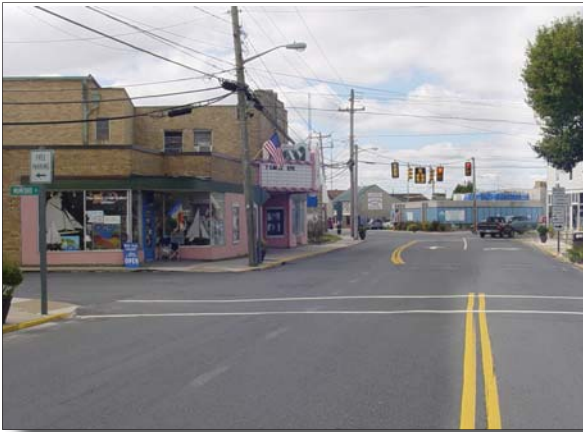
Existing Power Poles Along East Side of Main Street
