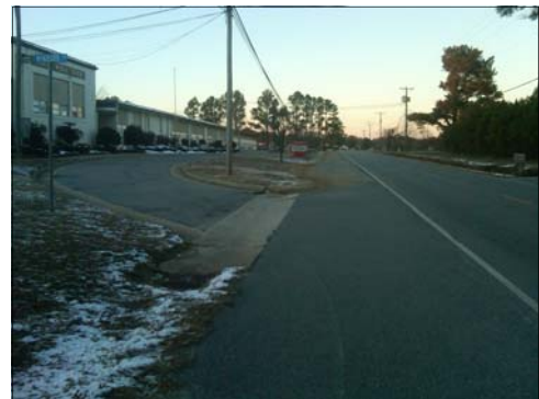
North Court Road in front of the school
